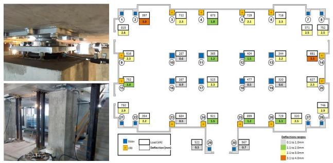
*Figure 10. a)* View of slider during jacking (left, top) b) Slider location atop column, shoring in place (left, bottom) c) Force-Deflection summary after load transfer complete.
