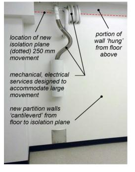
Figure 9. Illustration of basement wall and details to accommodate 250 mm movement at isolation plane.
