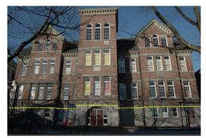
Figure 2. Basement, two storeys plus attic heritage classroom building; level of seismic isolation plane shown by dashed line.
